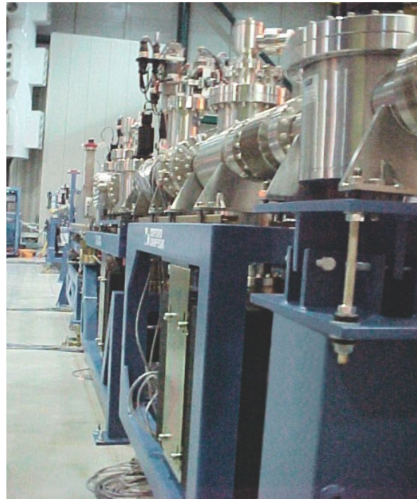
During installation of the GCPCC beamline at CAMD
